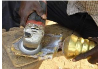
Figure 8: Grinding a brazed brass joint with a grinding disc accessory in an angle grinder. Source: Emeriewen, 2014.
